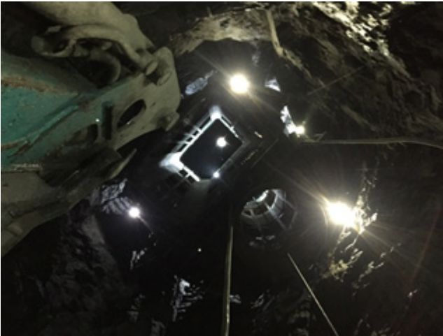
Exhibit 8: Central Shaft view from 326m below surface
